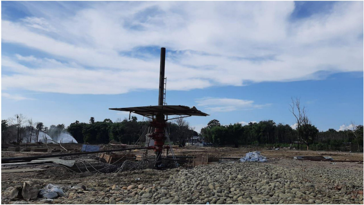
Baghjan well no 5 after successful diversion of flow of gas to nearby Early Production Setup (EPS)
